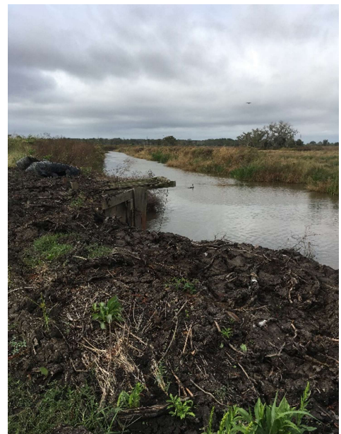
Figure 5 Water flap gate on Eastern side of North Unit, showing damage from Hurricane Michael, resulting in high water levels.
