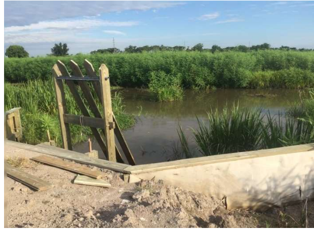
Figure 2 Rice Trunk 2, installed and functioning by August 1, 2019.
